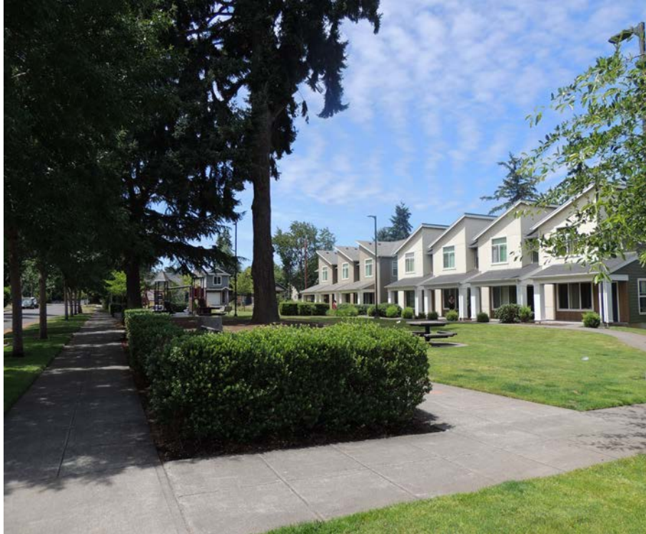
Mixed-income redevelopment in New Columbia apartments in Portland, OR helps to provide more affordable housing
